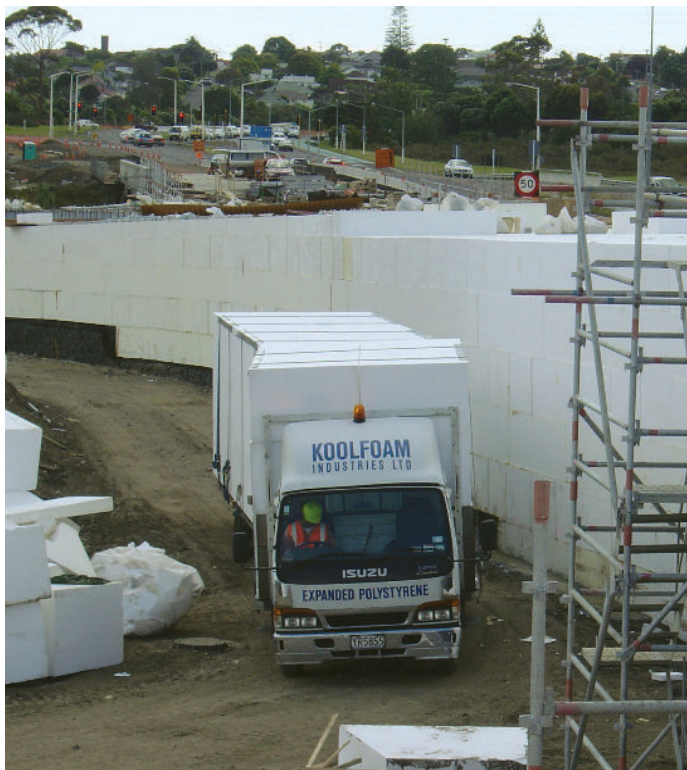
42,000m 3 Koolfoam Geofoam supplied for the Tauranga Eastern link project 2013 through 2015.
